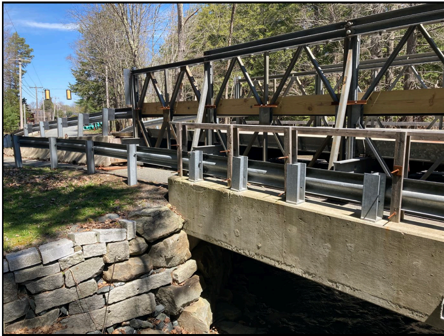
Figure 2: Cromwell Brook Bridge #3 Bridge (#0452)
